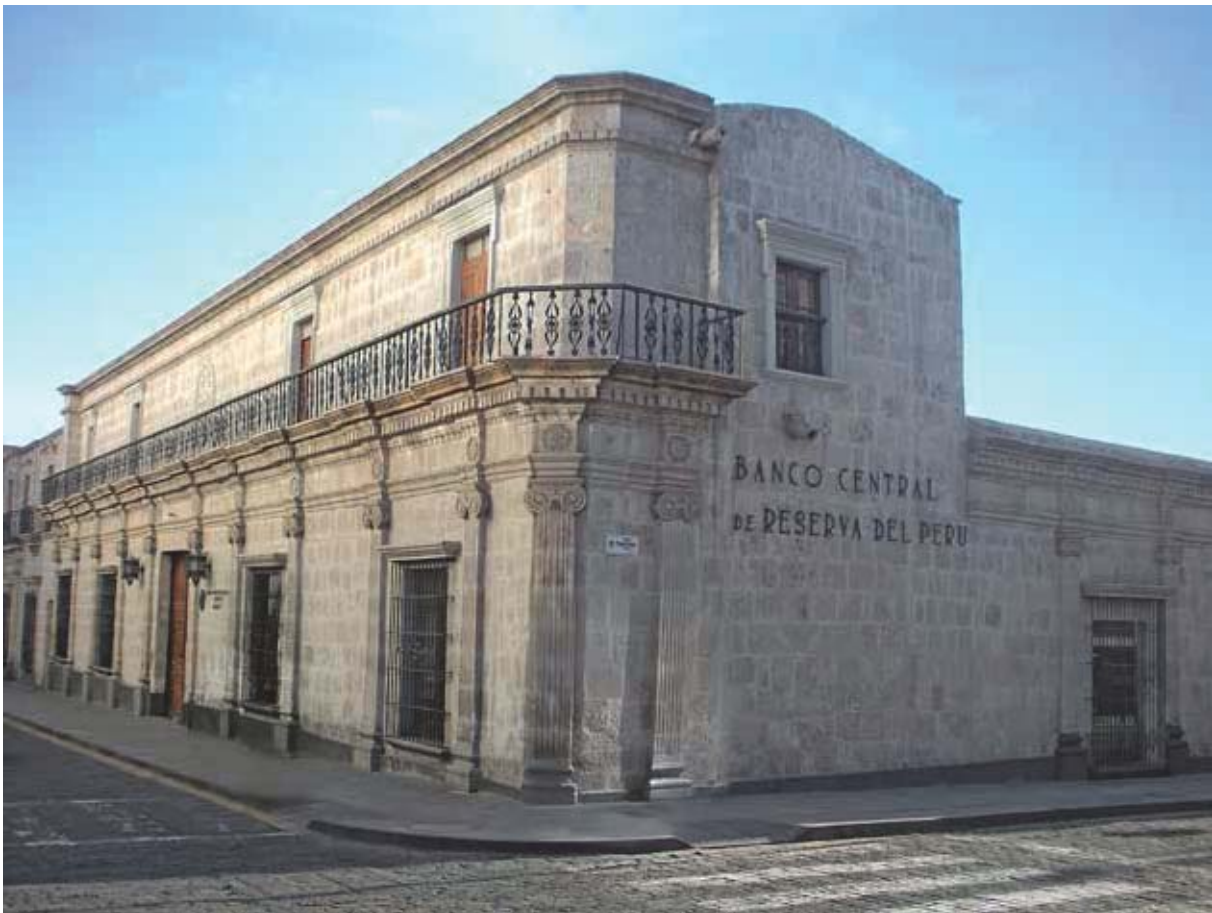
Façade of Casa Goyeneche, current building of the BCRP Branch Office in Arequipa.
