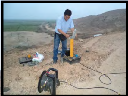
DATA RECORDER SLOPE INDICATOR.
